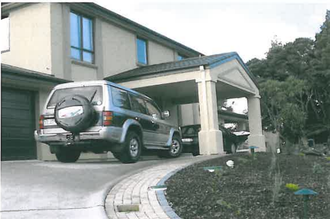
Figure 6. Blending the ProSTEP™ interceptor tank into the surroundings
